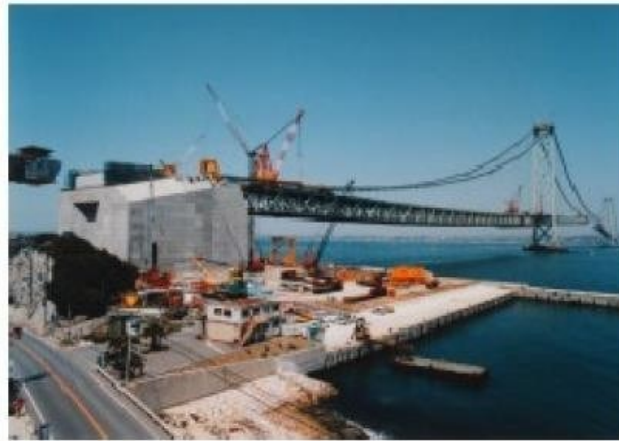
Anchorage 4A of Akashi-Kaikyo Bridge
